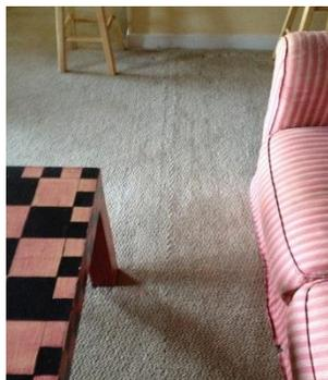
On the left is an installation issue. The installer placed a seam that runs perpendicular to the window. Any light coming through will magnify any changes of the height of the carpet. What you are seeing is both the height of seam tape as well as the seam itself.
